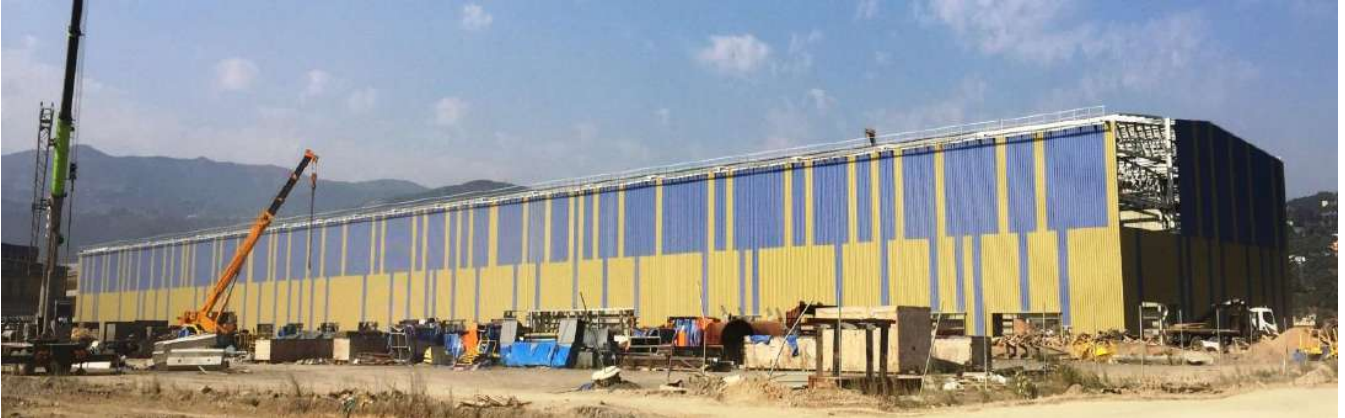
PK #11 – Wire Rod Warehouse: External side view for cladding works.
