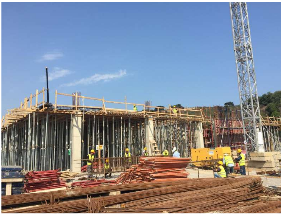
PK #02 – Mosque: Formwork and steel rebar for the slab 1 st level on-going.
