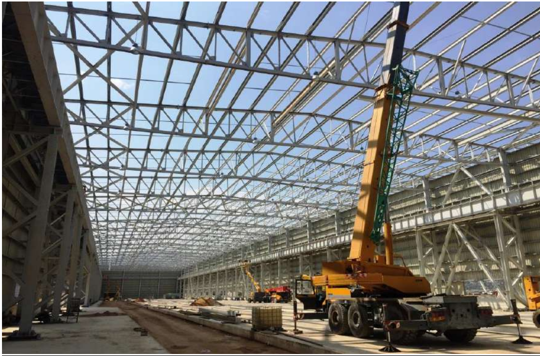
PK #11 - Wire Rod Warehouse:: Steel Structure erection and slab reinforcement (for train rail track) on-going
