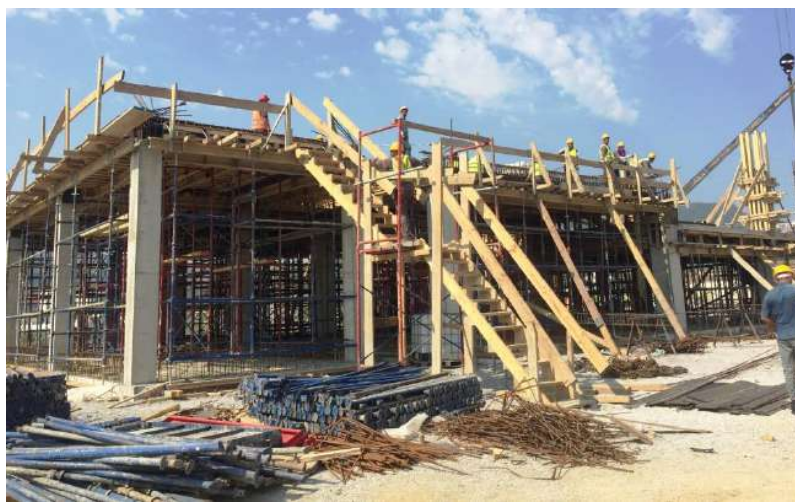
PK #02 – Mosque: Formwork and steel rebar for the slab 1 st level on-going.
